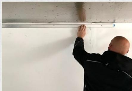
Aluminum Flashing/ Metal bar
