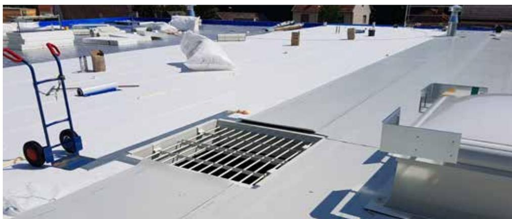
Approx. 2,300 m<sup>2</sup> pitched roof made of trapezoidal sheet metal as a supporting shell, self-adhesive vapor barrier / EPS thermal insulation, installed with staggered layers of adhesive / KÖSTER TPO 2.0 SK (FR) self-adhesive. An approx. 200 m<sup>2</sup> roof area with concrete slab has the same build-up.
